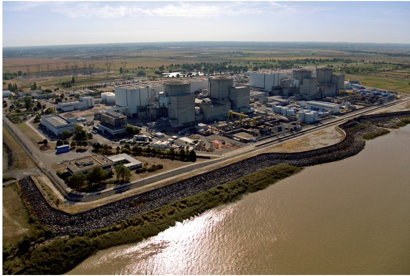
Figure 1.3: Aerial view of the Blayais nuclear power plant with its four production units and the protective dikes. Credit: Didier Marc.
